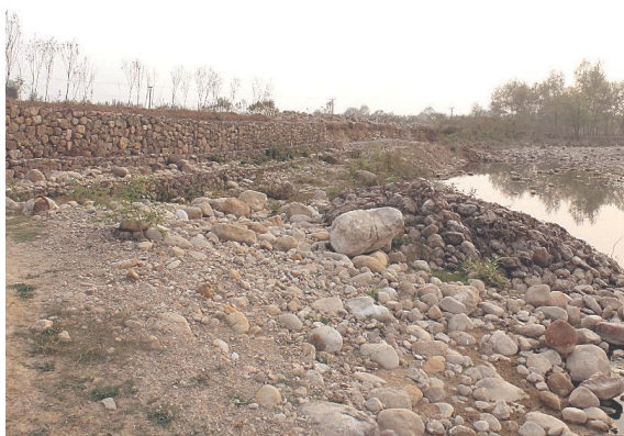
Figure: Gabbion constructed on Inguria river at Rupandehi
