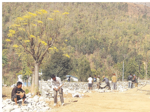
Mason training for earthquake resilient building construction
