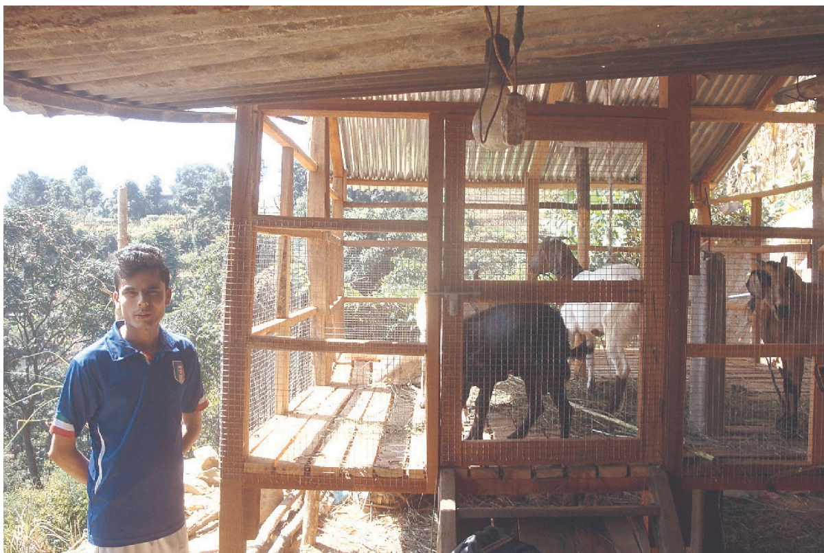
Figure: Improve shed construction at Kewalpur of Dhading district
